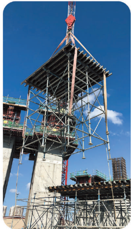
Hoisting Tableform at Razer S.E.A Headquarter
