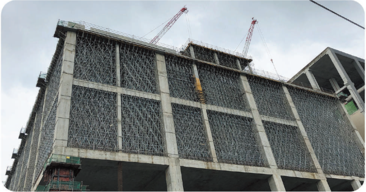
Logistic centre at 47 Jalan Buroh
